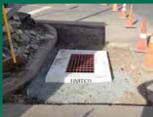
Catch Basin Installation
